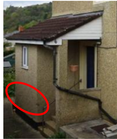
S38 – 6 Upper Park Road, Nailsworth. Side extension (in blockwork) & porch
