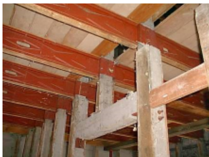
TYPICAL PARTY WALL Finishes removed showing columns
