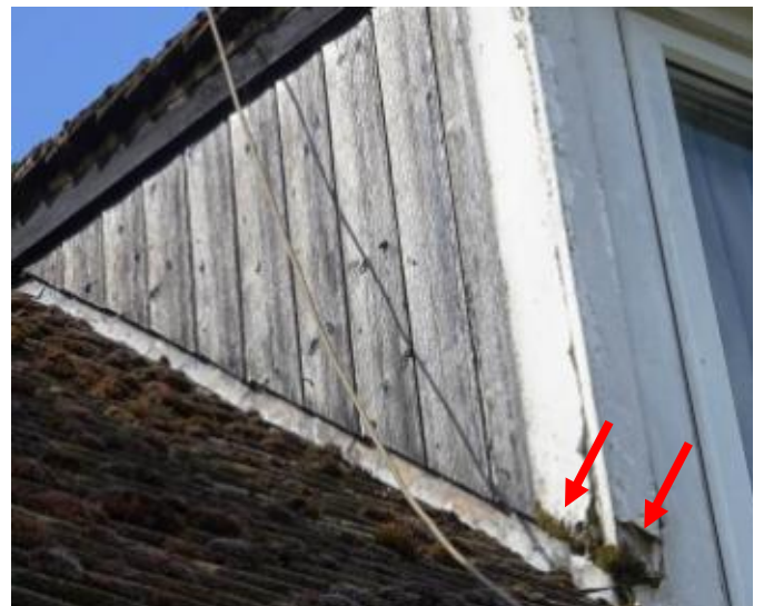
T40 – 7 Mount Pleasant, Wotton-Under-Edge. Rear, poor timber to dormer side, and architrave rotten near roof tiles (arrowed)
