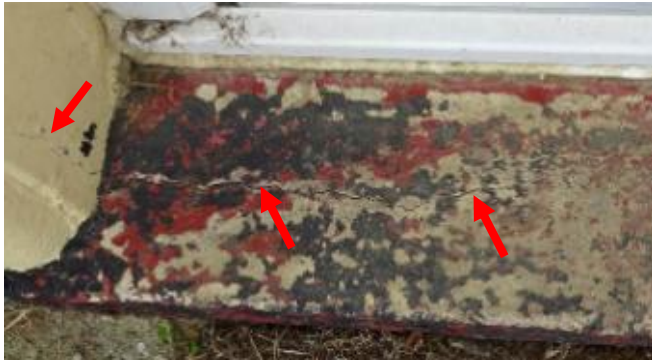
S31 – 51/52 Mankley Road, Leonard Stanley. Crack on door step extending up onto reveal
