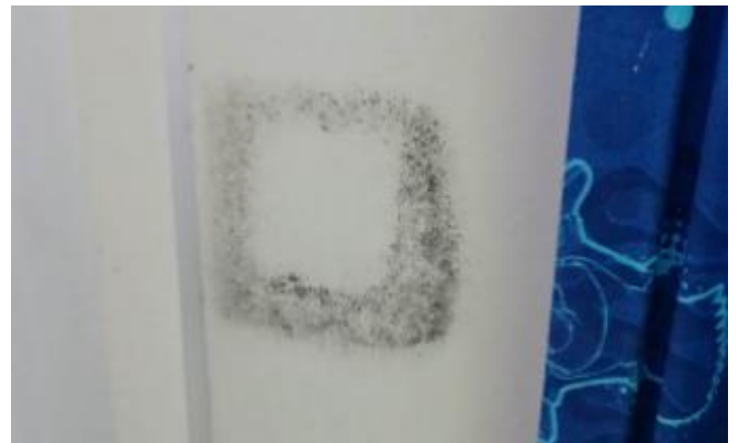
S20 – 12A Lawnside, Forest Green, Bedroom mould to left of window mid height
