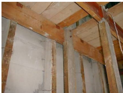
TYPICAL PARTY WALL Finishes removed showing columns
