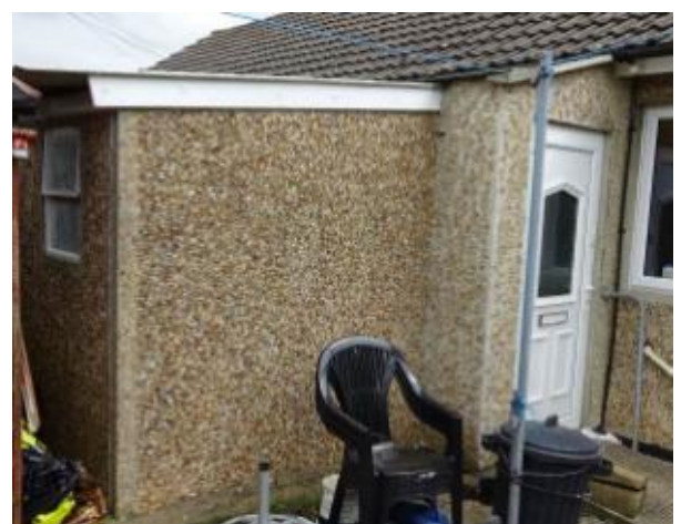
S36 – 38 Glebe Road, Minchinhampton. Outbuilding of Reema panel construction jointed to bungalow
