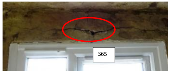
S62 – 31 Victory Road, Whiteshill. Side extension cracking above window (S63 circled)
