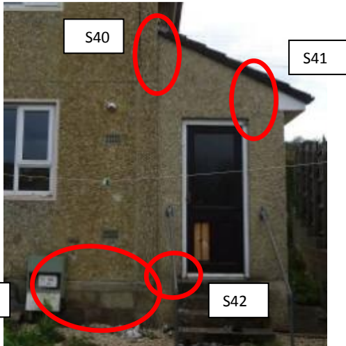
S39 – 6 Upper Park Road, Nailsworth. Side extension from rear
