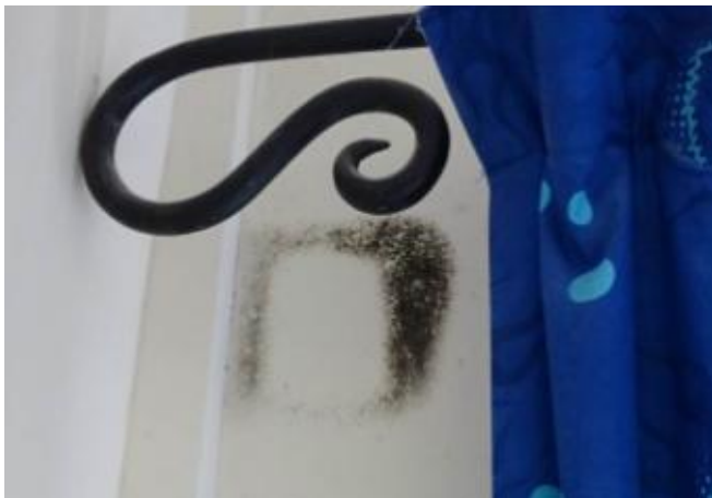
S19 – 12A Lawnside, Forest Green, Bedroom mould to left of window high level
