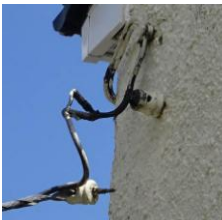
P11 – Overhead power supply fixing at wall, at 14 Hyett Road, Cashes Green
