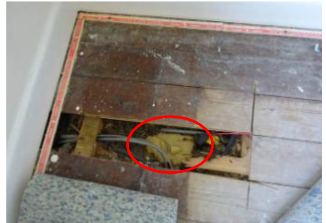
S46 – 3 Upper Park Road, Nailsworth. First floor construction (S47 circled)
