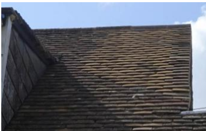
T35 – 3 Mount Pleasant, Wotton-Under-Edge. Gable chimney taken down
