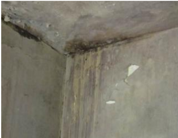
S69 – 31 Victory Road, Whiteshill. Side extension mould & damp ingress staining in front corner
