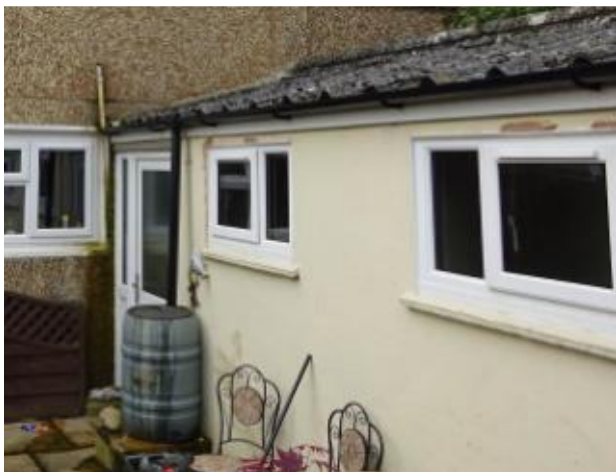
S59 – 26 Willow Road, Stonehouse. Outbuilding joined to the bungalow (note: Outbuilding is blockwork construction)
