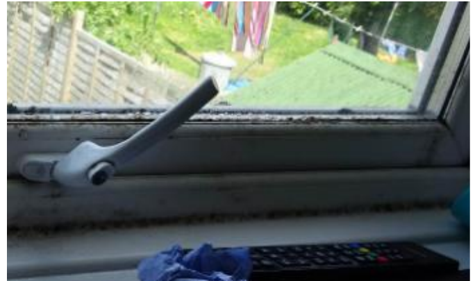
P8 – 14 Mosley Cresnet, Cashes Green, mould on window frame in rear bedroom
